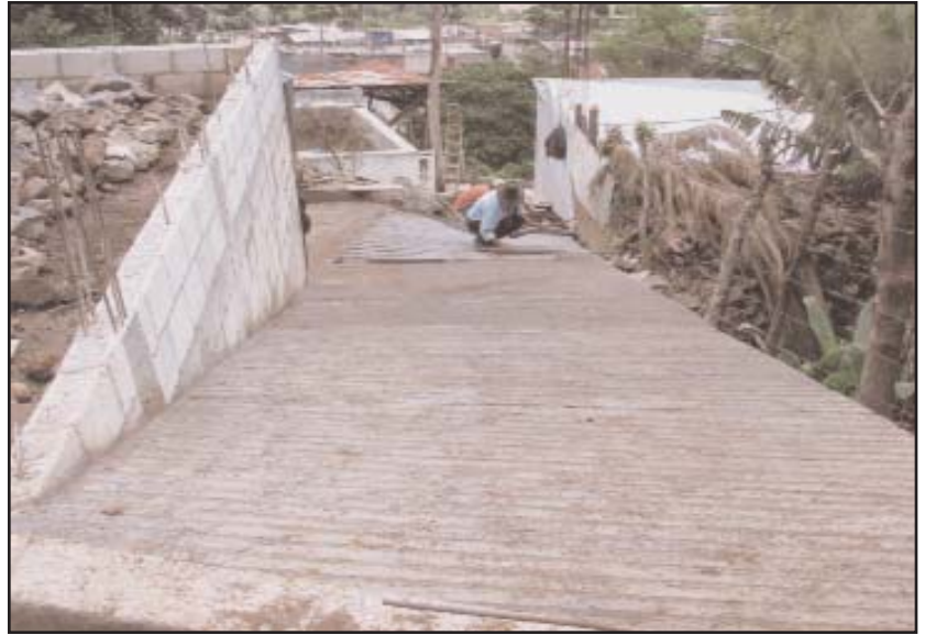
A long ramp had to be built ...
