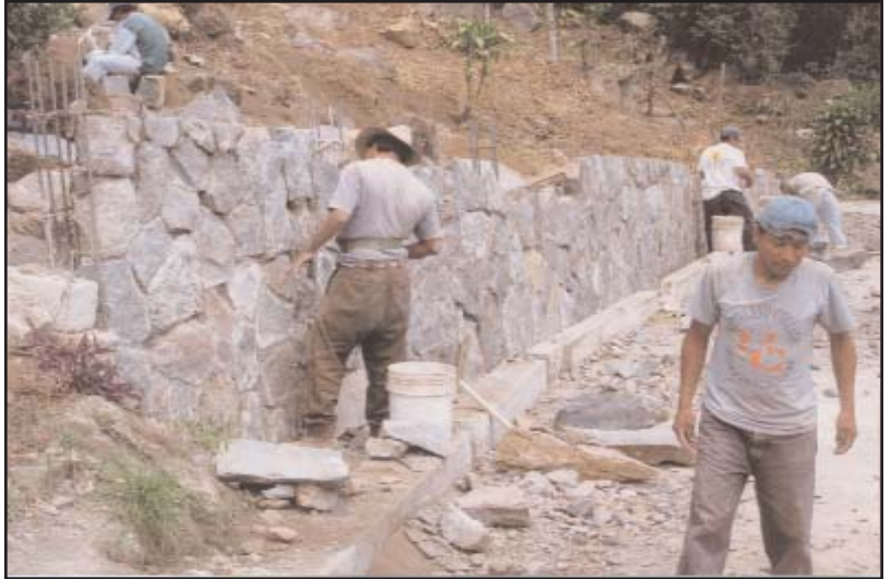
Retaining walls had to be built...
